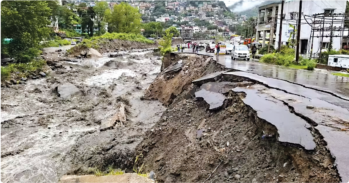
Figure 21: Disruption in pilgrimage movement during Manimahesh yatra due to floods and landslides in Chamba district.
