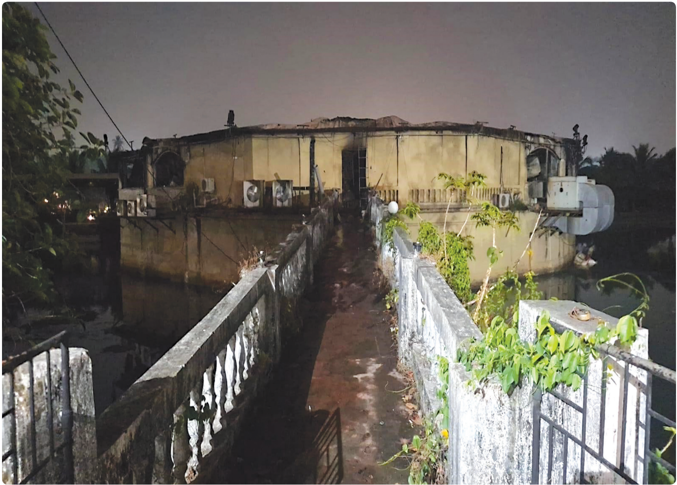
Figure 75: The first-floor exit opens onto a narrow bridge on two sides, the front and rear, and is surrounded by khazans – low-lying lands used for agriculture and aquaculture – near the Baga River.
