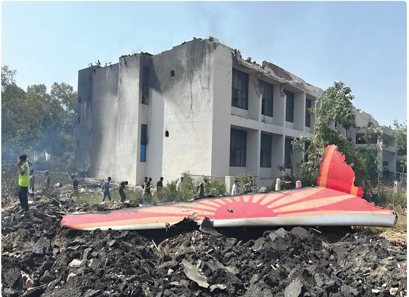
Figure 2: Post-crash wreckage of the Air India Dreamliner and structural damage to the adjacent hostel building at the impact site.
